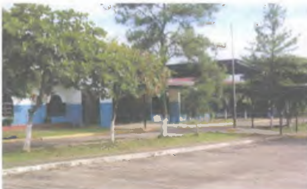
Figura N° 20 Hospital Regional de Chepo
