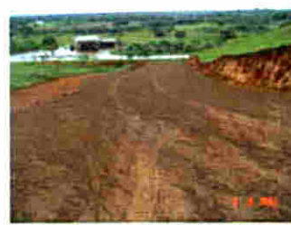
View from Top of Road (looking East)
